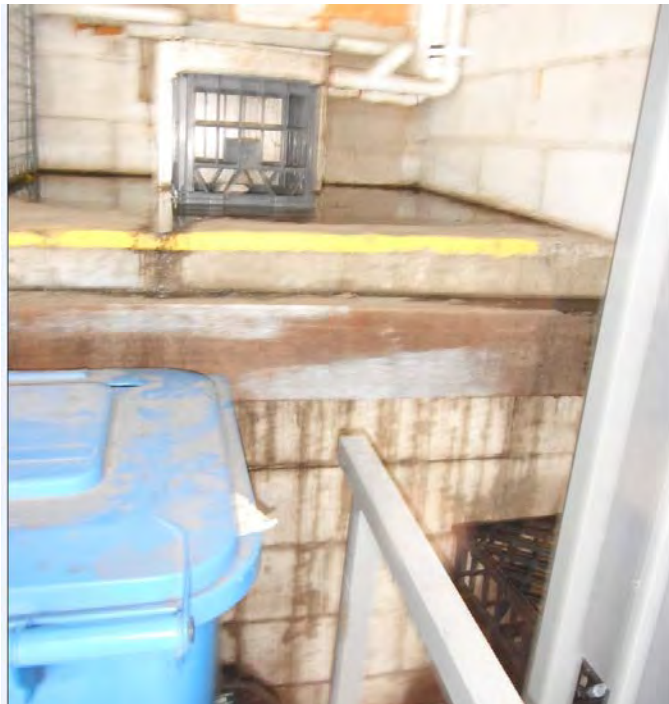
Photo 3 – Overflow of waste water filter system leaking below the raised concrete platform
