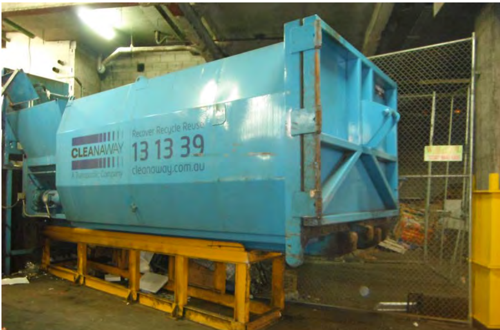
Photo 6 – Cardboard compactor observed in the loading dock area of Burwood Plaza
