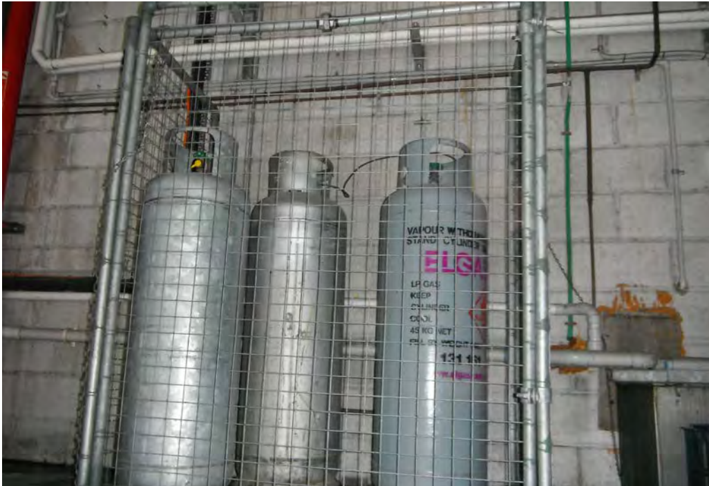
Photo 1 – Three LPG gas cylinders stored in the metal cage located in the loading dock area of Burwood Towers
